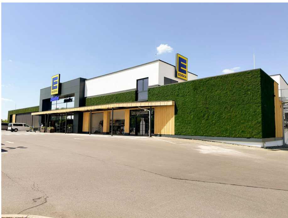
MARKET FAÇADE · ENTRANCE
