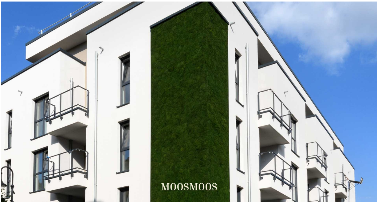
FINISHED MOSS FAÇADE · TWO AND A HALF YEARS AFTER INSTALLATION
