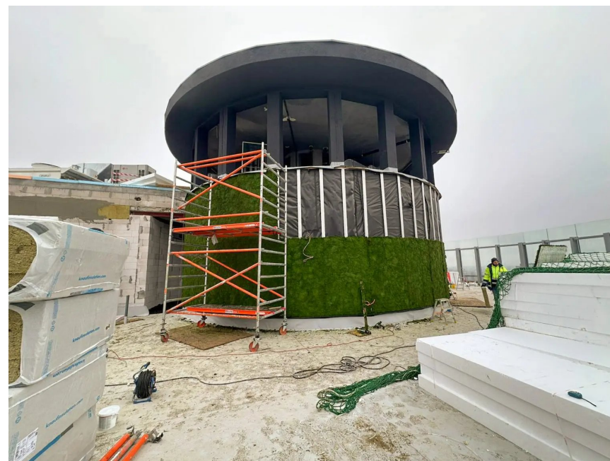
INSTALLATION AT AN EXPOSED HEIGHT
